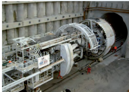
Figure 4: Gripper TBM after refurbishment ready to be used for the Erstfeld contract of the Gotthard tunnel after completing the Amsteg section of the Gotthard tunnel.
